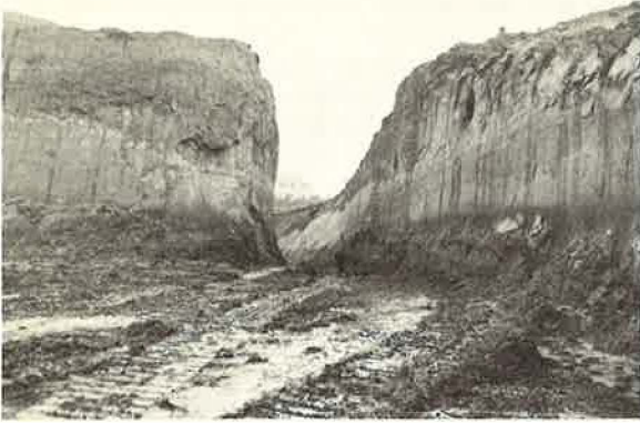
Figure 3. An example of a relatively stable vertical cut in loess. This particular cut is in a gravel pit in Tipton County. It is approximately 25 ft in depth.
