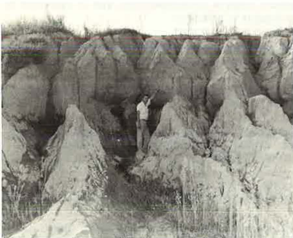
Figure 2. An example of the highly erosive nature of loess. These slopes had originally been constructed on a 2:1 slope ratio and had gone unattended for approximately 18 months.
