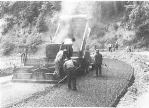
Figure 7. Placing open-graded asphalt-concrete drain layer.
