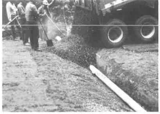
Figure 6. Placing open-graded asphalt-concrete drain material around pipe.
