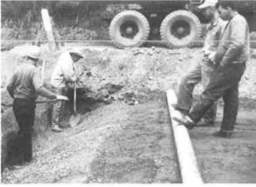
Figure 5. Placing filter material in transverse trench.
