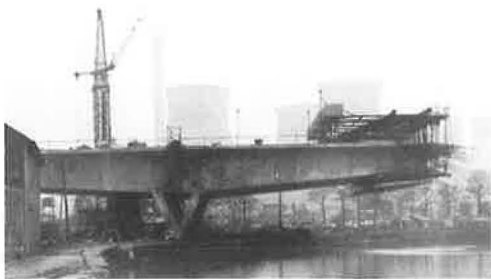
Figure 8. River Aire Bridge—south cantilever.
