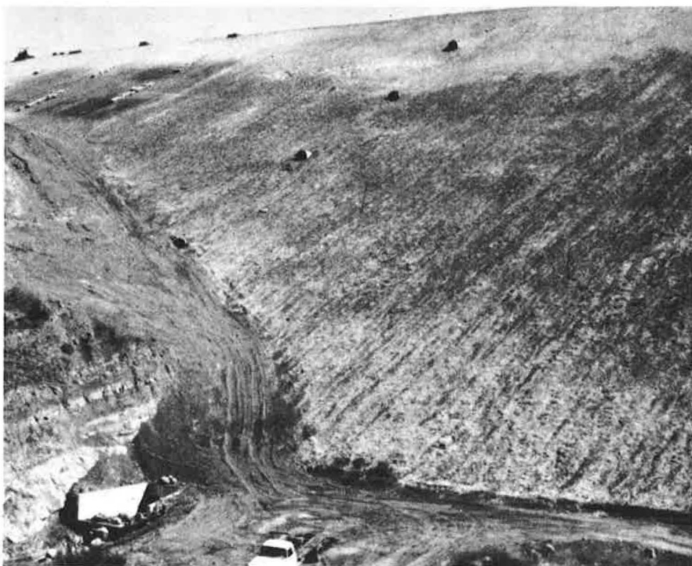
Figure 13. Side of embankment on Ridge Route showing the instrument shelters.
