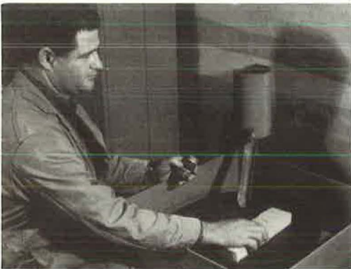
Figure 5. Grinding exposed surface with silicon carbide abrasive.
