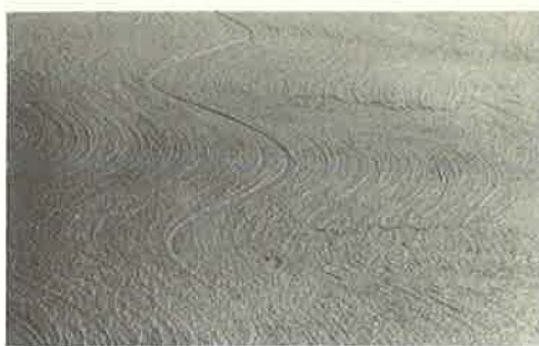
Figure 12. Natural texturing by longitudinal wooden float.
