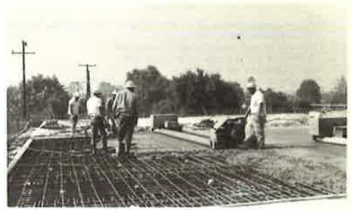
Figure 6. Clarey strike-off machine.
