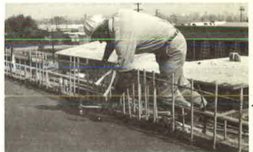
Figure 18. Placing grid reference points.
