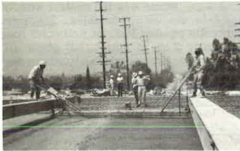
Figure 7. Sixteen-foot longitudinal plow handle float.
