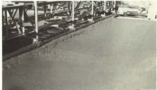
Figure 4. Trueline strike-off machine.
