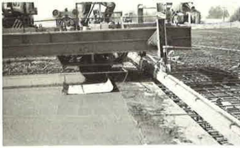
Figure 5. Borges strike-off machine.
