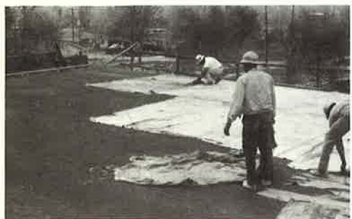
Figure 13. Placing rugs for a wet rug cure.
