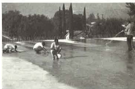
Figure 26. Conducting a deck crack survey.
