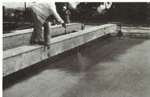
Figure 14. Applying liquid membrane-type curing compound.
