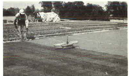
Figure 10. Surface texturing with stiff bristle broom.
