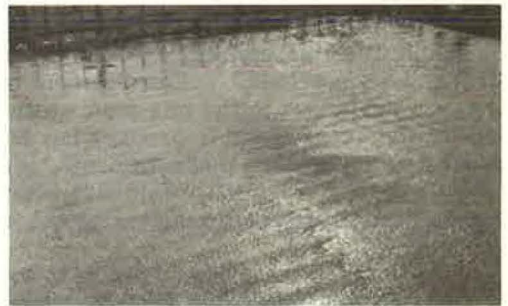
Figure 20. Excessive bleed water.
