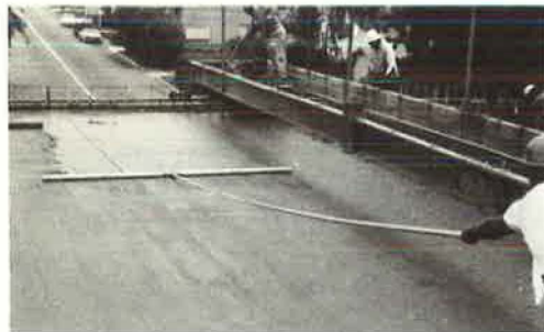
Figure 9. Aluminum float (4-in. diameter, 10 ft long) with handle.
