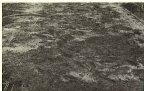
Figure 21. Excessive walking in the fresh concrete.
