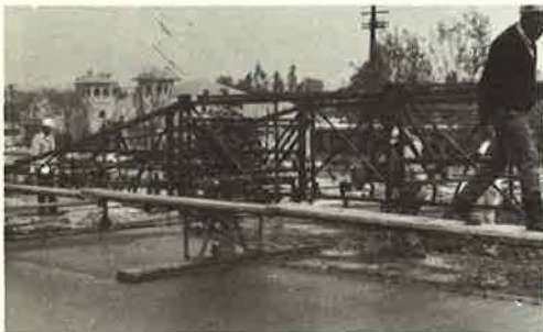
Figure 3. Bidwell strike-off machine.
