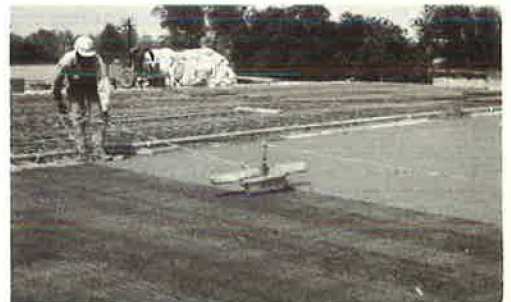
Figure 10. Surface texturing with stiff bristle broom.
