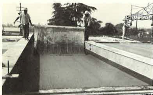
Figure 11. Surface texturing with burlap drag.
