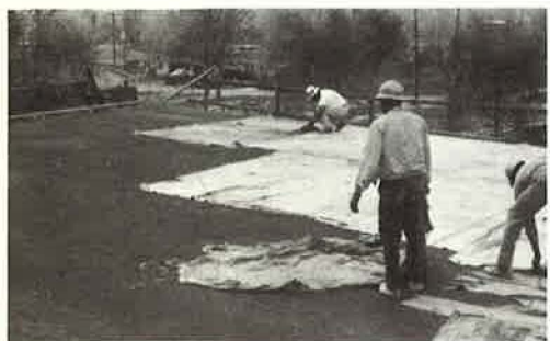
Figure 13. Placing rugs for a wet rug cure.
