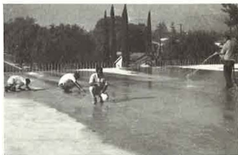
Figure 26. Conducting a deck crack survey.
