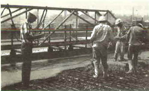
Figure 19. Recording concrete placement.
