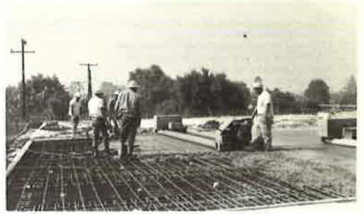
Figure 6. Clarey strike-off machine.
