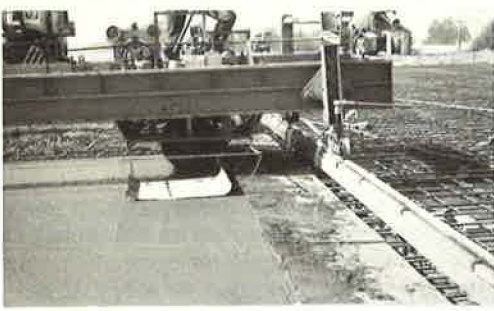
Figure 5. Borges strike-off machine.
