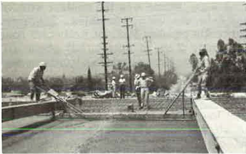
Figure 7. Sixteen-foot longitudinal plow handle float.
