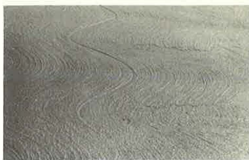
Figure 12. Natural texturing by longitudinal wooden float.
