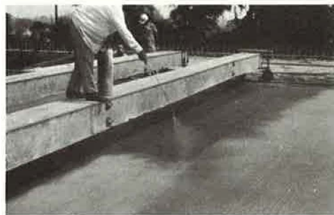
Figure 14. Applying liquid membrane-type curing compound.
