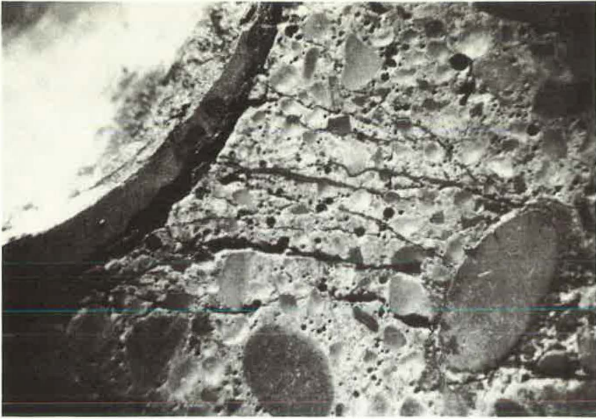
Figure 9. Shattered paste resulting from steel corrosion (mag. 12X).
