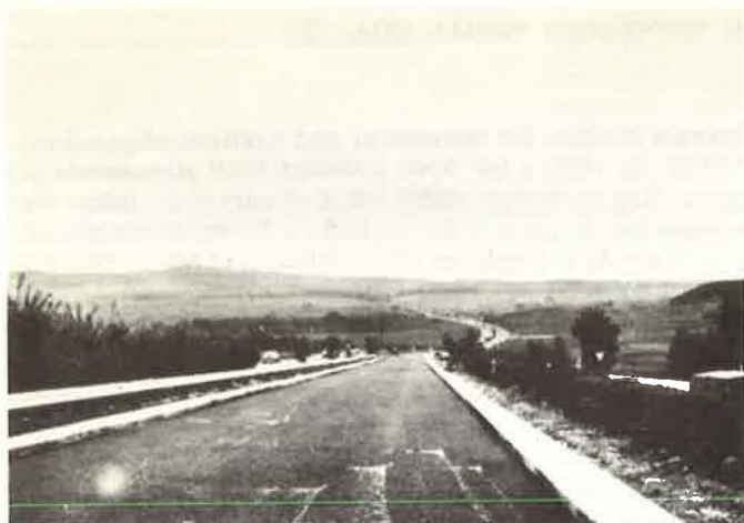
Figure 1. A winding alignment visible over a considerable length appears artificial unless the natural features responsible for the curvature are visible.
