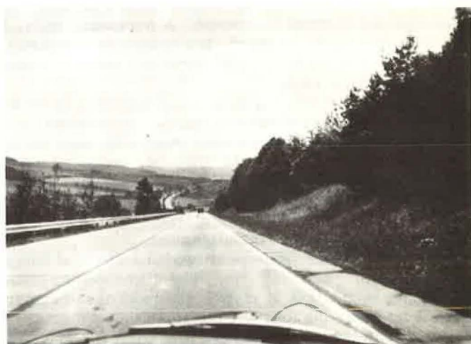
Figure 2. An example of sight loss and a poor combination of vertical curvature.
