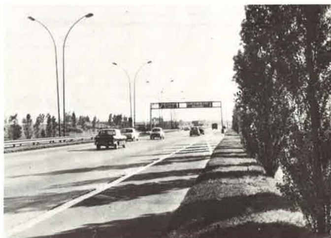
Figure 6. Poor visibility at a fork: in this case, the minor fork is on the left (this disposition should never be adopted); the straight, horizontal alignment hides the fork, which only appears at the last moment for a driver who is not concentrating.
