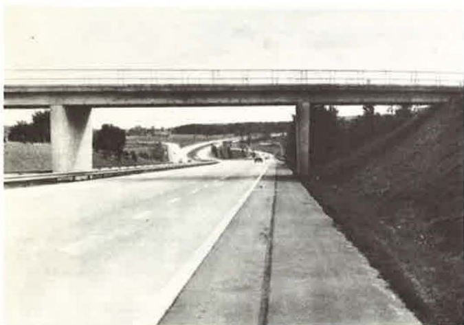
Figure 5. The same fork (farther on): the exit ramp aligned with the previous roadway seems to be the main road, while the main road is hidden by an inflexion on the left and is nearly invisible—the driver can be misled by the appearance of the exit into making dangerous maneuvers.
