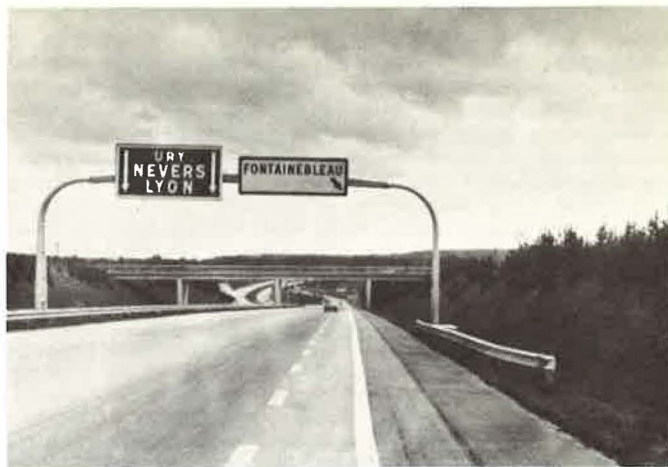
Figure 4. Sight loss near a fork: the driver cannot see the decision point shown by the signposting; this visual defect gives him a feeling of insecurity.
