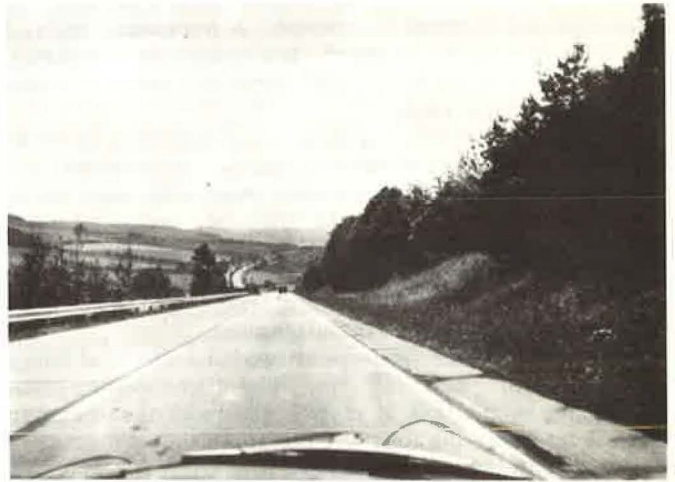
Figure 2. An example of sight loss and a poor combination of vertical curvature.
