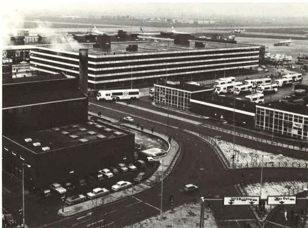
Figure 5. Car Park No. 3, Central Terminal area, London Heathrow Airport.
