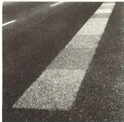
OVERALL VIEW OF AUBURN TEST SECTION AFTER 6 DAYS OF TRAFFIC
