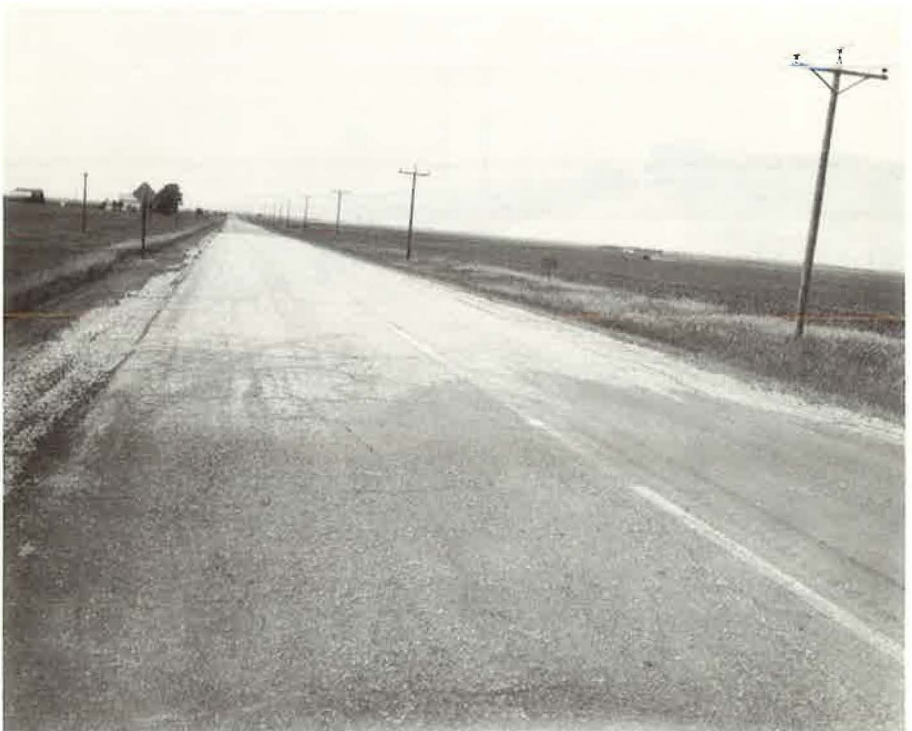
Figure 8. RC-4 with styrene-butadiene rubber, June 28, 1967.
