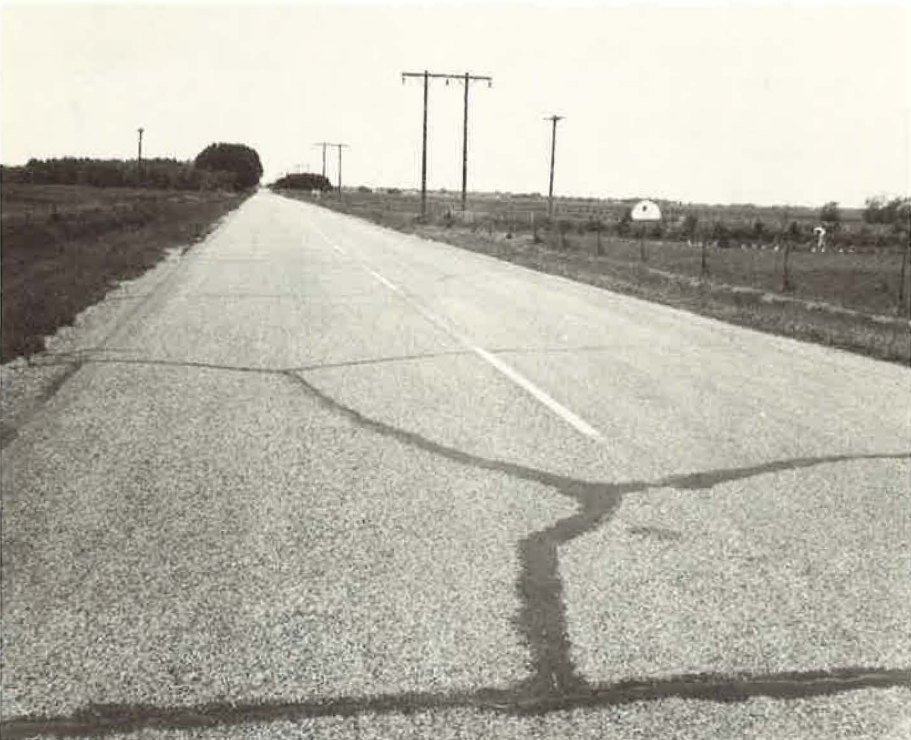
Figure 6. RC-4 with neoprene rubber, June 28, 1967.
