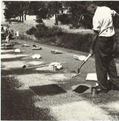
SPREADING AND INITIAL ROLLING OF SCREENINGS
