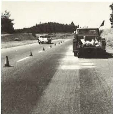
FINAL COMPACTION WITH A LIGHT DUTY TRUCK
