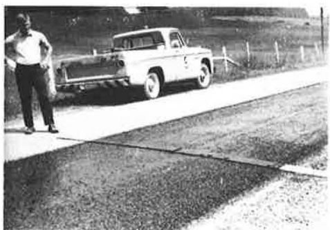
Figure 3. Cotton pad test strips being used to measure lateral distribution.
