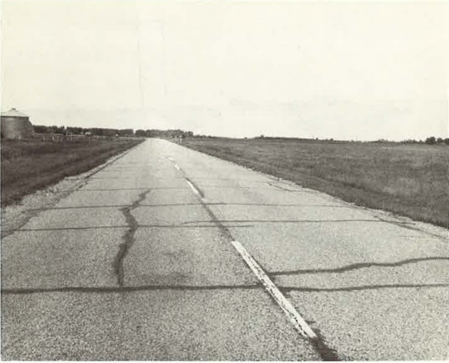
Figure 5. RC-4 with no-strip additive, June 28, 1967.
