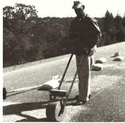
SPREADING AND INITIAL ROLLING OF SCREENINGS
