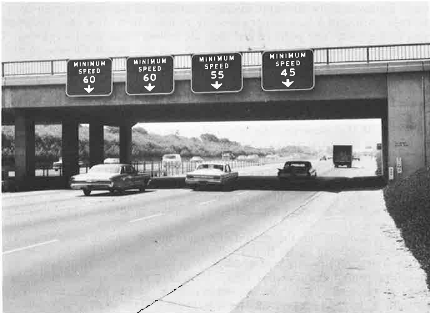
Figure 2. Placement of minimum speed signs on 8-lane freeway.
