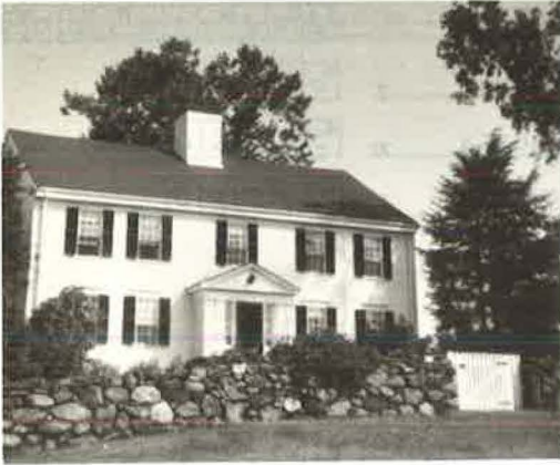
Figure 4. Photograph of the Kimball-Rowe-Allen House.
