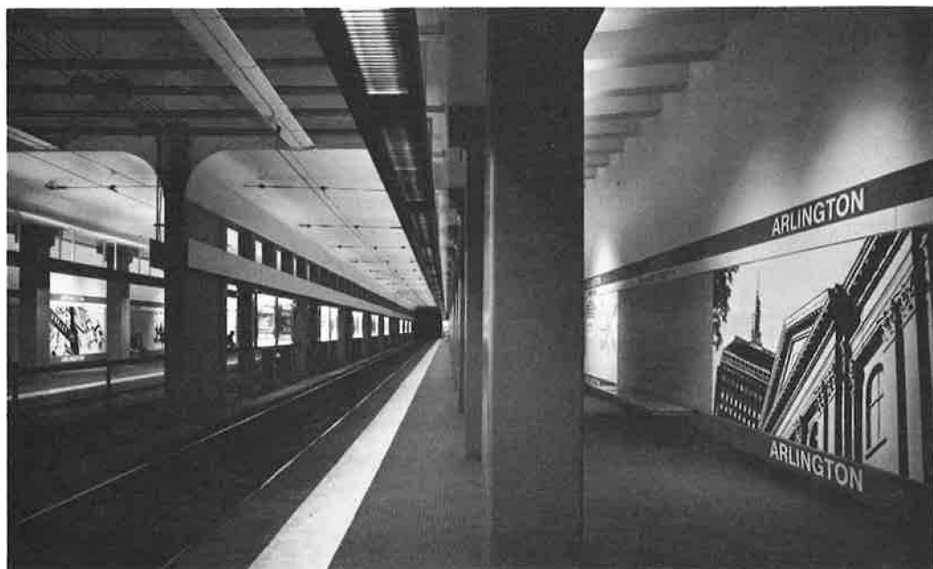
Figure 6. Remodeled station platform, showing walls facing the trains, with name bands, directional signs and photomurals, and showing center track area, facing the waiting passenger, with advertising posters.
