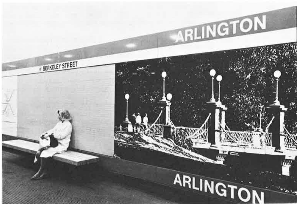
Figure 5. Segment of side wall at remodeled platform, showing upper and lower color-coded name bands, white directional sign band, map and typical photomural.
