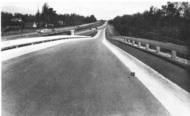
Figure 8. Metal plate (left) and metal beam (right) guardrail.
