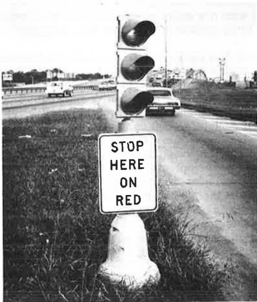
Figure 5. Ramp control signal used on the Gulf Freeway.
