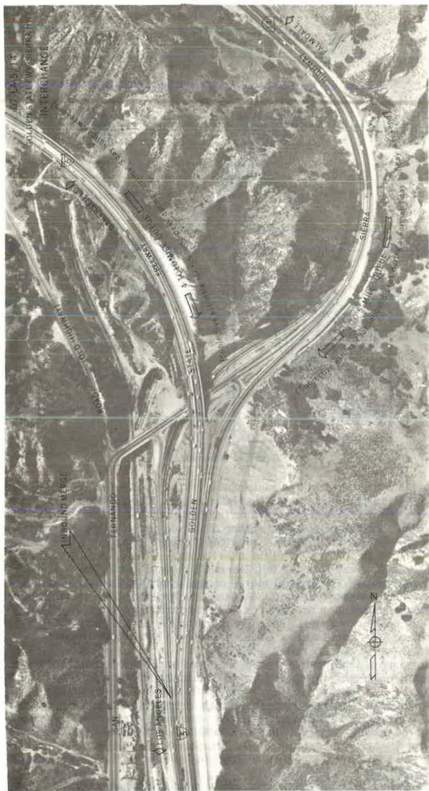
Figure 2. The Golden State Freeway and Sierra Highway interchange.
