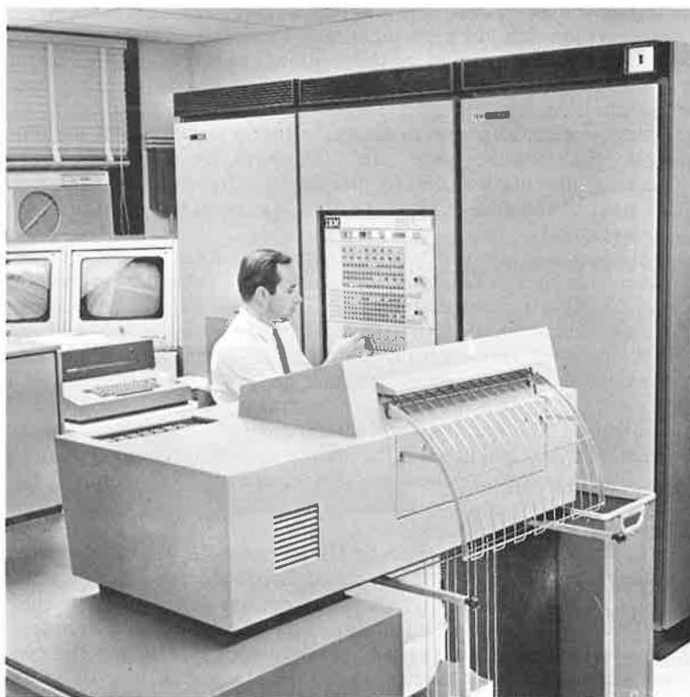
Figure 9. IBM 1800 digital computer in Gulf Freeway surveillance and control office.
