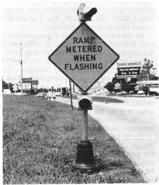
Figure 6. Advance warning sign used on the Gulf Freeway.
