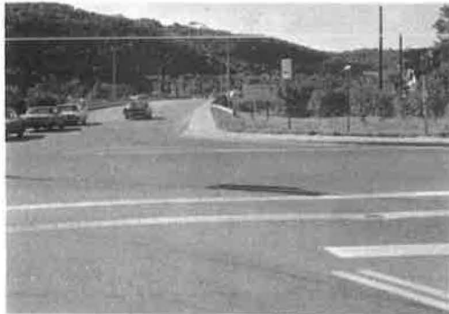
Figure 17. Landscaped approaches, Bevier Street Bridge.
