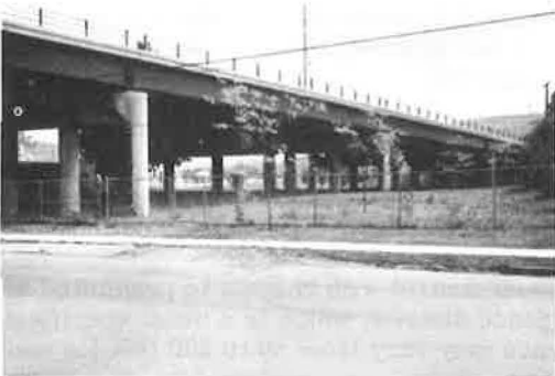
Figure 7. Under-structure parking area, urban arterial.
