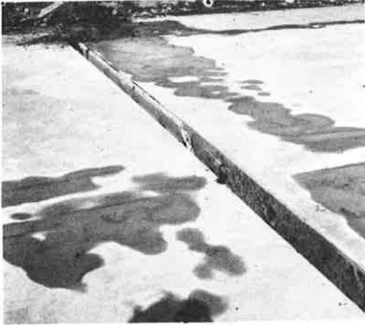
Figure 3. Joint 3—sawed face of slab III showing the steel collars.
