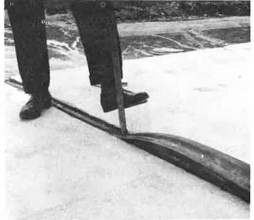
Figure 4. Placing seal in joint 1.
