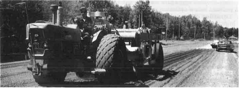
Figure 18a. In-place mixing of salt and aggregate on the Ontonagon project.
