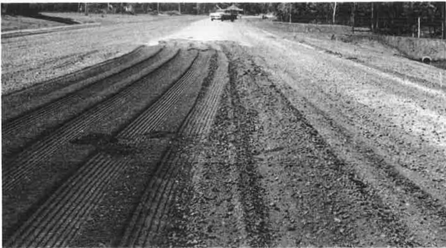
Figure 18b. Salt-treated base after mixing (unmixed salt in background).
