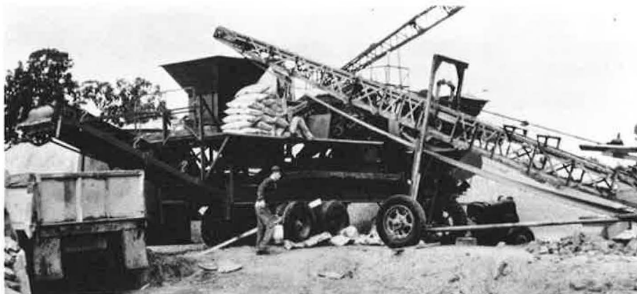
Figure 4a. Pug mill for mixing aggregate, fines, and salt.
