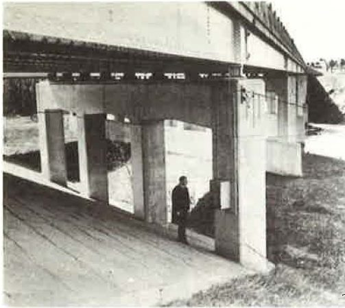
Figure 5. Location of the power supply and control center on the Flint River bridge application on I-75.
