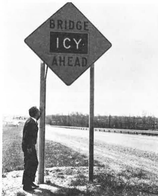
Figure 2. Electric flasher that warns of icy conditions on highway overpasses and bridges.
