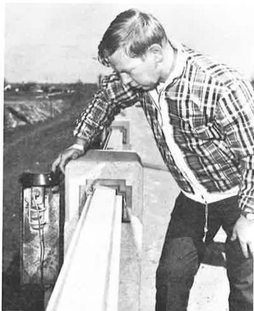
Figure 3. Location for the temperature- and humidity-sensor unit on a bridge railing.
