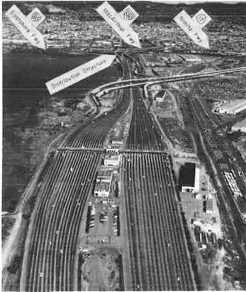
Figure 3. San Francisco-Oakland Bay Bridge Toll Plaza (looking east).
