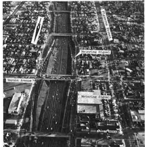
Figure 8. Vernon Avenue on-ramp where single-car metering from 2 lanes is used because of limited storage space. Metering signals are used on the 1-way frontage road to keep stored traffic from blocking the Vernon Avenue intersection. Green phases of the frontage road and Vernon Avenue signals coincide. Queue on the northbound off-ramp is unrelated to project; queues were a frequent occurrence before controls.
