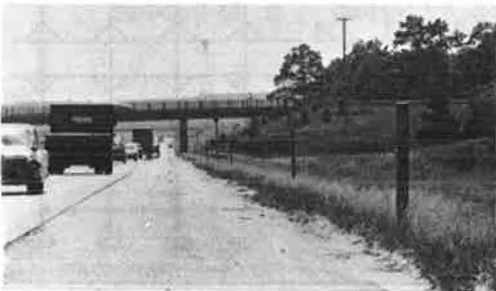
Figure 4. Typical installation of roadside detector.
