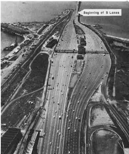
Figure 2. San Francisco-Oakland Bay Bridge Toll Plaza (looking west).
