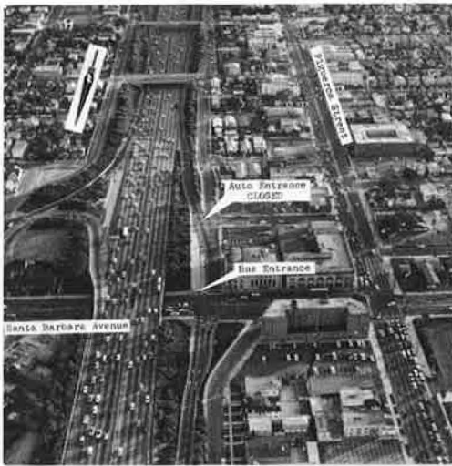
Figure 7. Santa Barbara Avenue on-ramp that is closed because of lack of storage space. Buses have always had a separate entrance to the ramp and can be easily allowed special access. Ramp is closed by hand-placed barricades that will be eventually replaced by automatic "pop-ups". Queue on Figueroa Street is the result of preferential signal timing for Santa Barbara Avenue traffic. Although not related to the project, green time on Santa Barbara Avenue has been increased since the start of controls. This is the key intersection in the entire project area.
