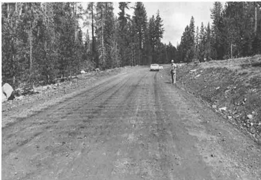
Figure 1. Sycan Road, North of Bly, Oregon: Note contrast between washboard surface using purple cinders (foreground) and smooth surface using red cinders (background).
