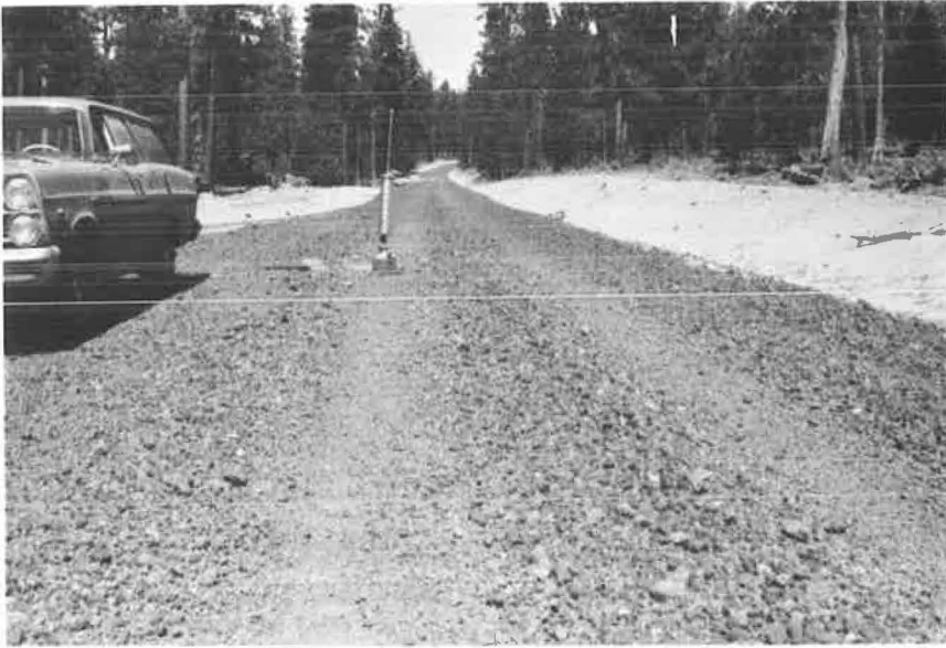
Figure 2. Kirk Road, Northeast of Chiloquin, Oregon: Rough surface contains black, uniformly graded cinders (PI = 2.1).
