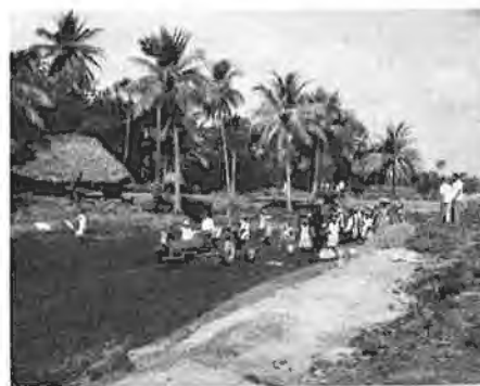
Pulverized black cotton soil being carried by the laborers
