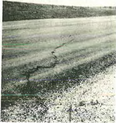
Figure 26. Cracks that developed in areas of bentonite soil.
