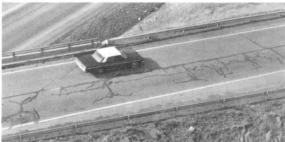
Figure 3. An oblique depicting pavement conditions in the later part of May 1967, a few days prior to the date of the multiple vertical coverages shown in Figure 1. The width of the sealant stripe is indicative, to a degree, of the severity of the pavement failure.
