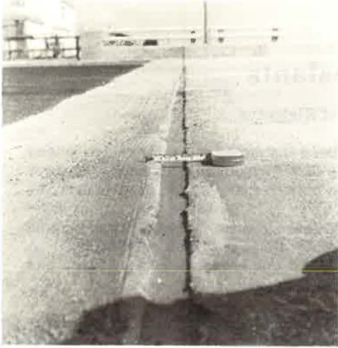
Figure 1. Formed joint groove.
