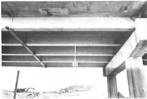
Figure 4. System 15—Linseed oil-alkyd red lead primer, traffic paint barrier coat, and vinyl primers and vinyl finish coat.
