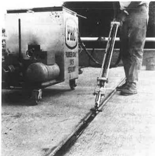
Figure 6. Polyurethane sealant.
