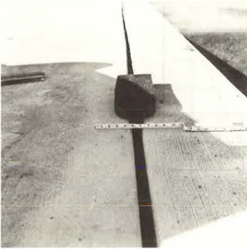
Figure 9. Asphalt-impregnated polyurethane foam.
