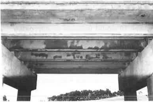
Figure 2. System 16—100 percent solids epoxy coating after 3 years of exposure; photo taken in 1961.
