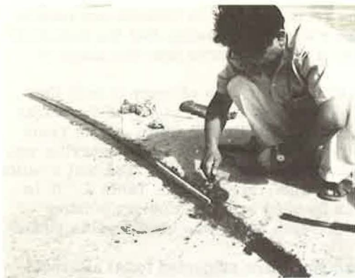
Figure 1. Preparation of central groove in the freshly laid resin sand mortar along a crack under repair on National Highway 2.
