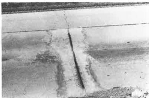
Figure 30. Expansion joint installed on I-59 in Jones County.
