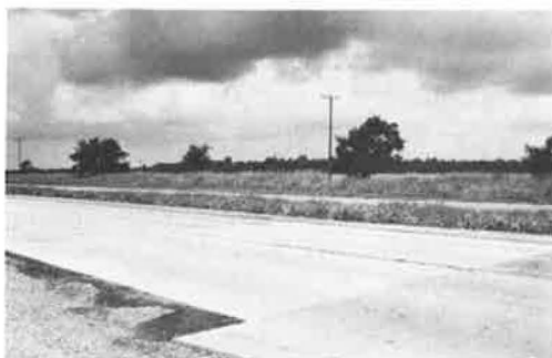
Figure 36. Complete patch 3 months after repair on US-82 in Leflore County.
