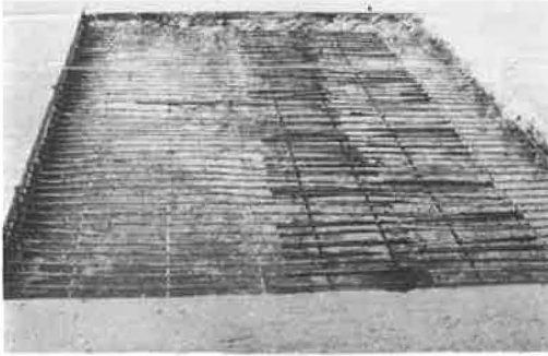
Figure 32. Patch ready for replacing concrete on I-55 in Madison County.
