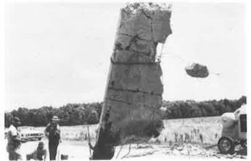
Figure 35. Investigation during repair on US-82 in Leflore County.
