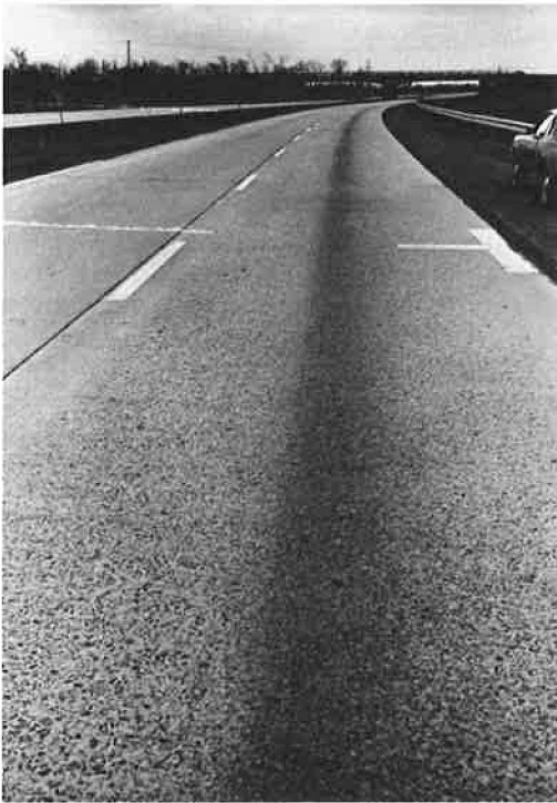
Figure 3. Studded tire wear on concrete pavement (Highway 17, Queensway, Ottawa, 6 years old, AADT 10,000 per lane).
