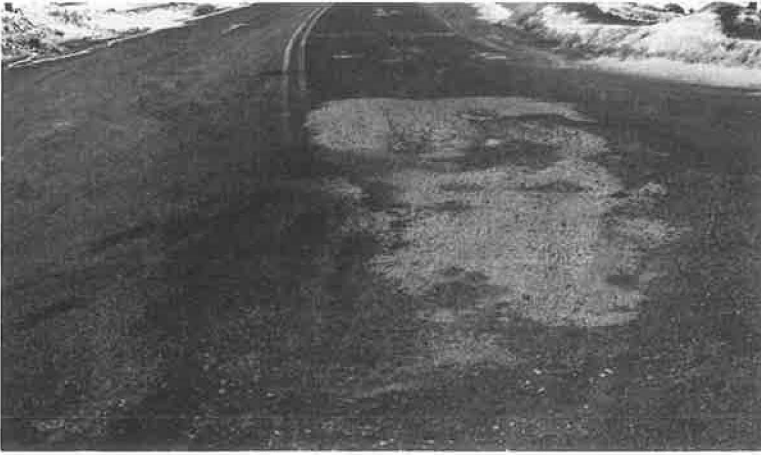
Figure 4. Localized wear at an intersection where vehicles stop, start, and turn.
