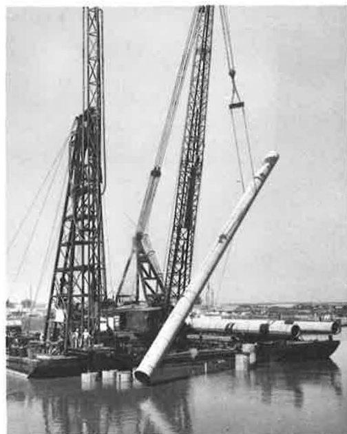
Figure 2. Prestressed concrete cylinder pile used in Napa River.
