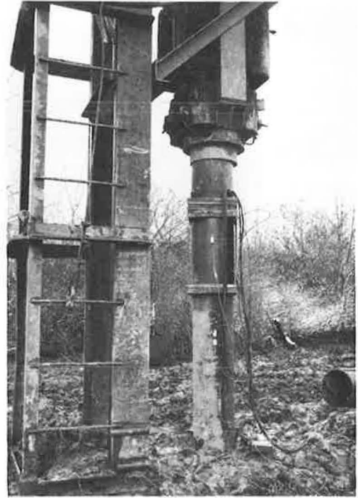
Figure 5. Force transducer and accelerometer in driving system.
