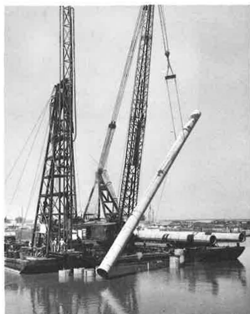
Figure 2. Prestressed concrete cylinder pile used in Napa River.
