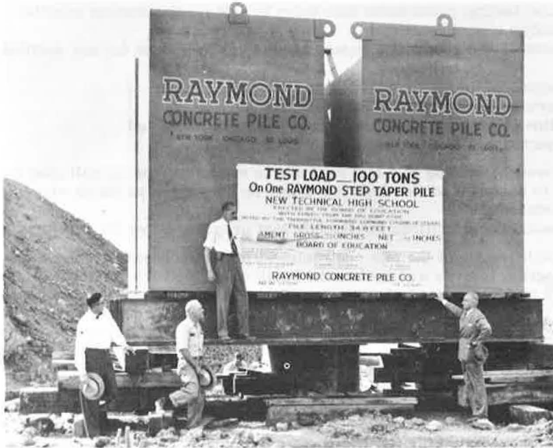
Figure 1. Test load applied directly to pile by using loaded platform and water-filled interconnected steel tanks.
