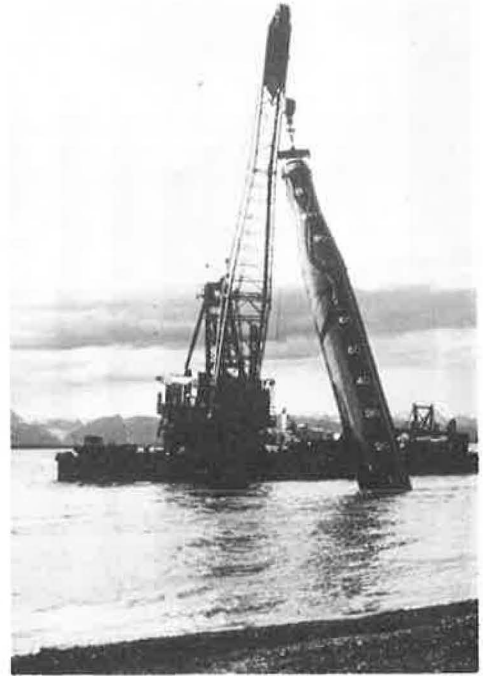
Figure 4. Steel caisson pile used in Cook Inlet, Alaska, to withstand vertical and horizontal loads.
