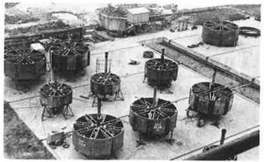
Figure 2. Bit bodies for Dutch rotary reaming 26-ft diameter mine shafts.
