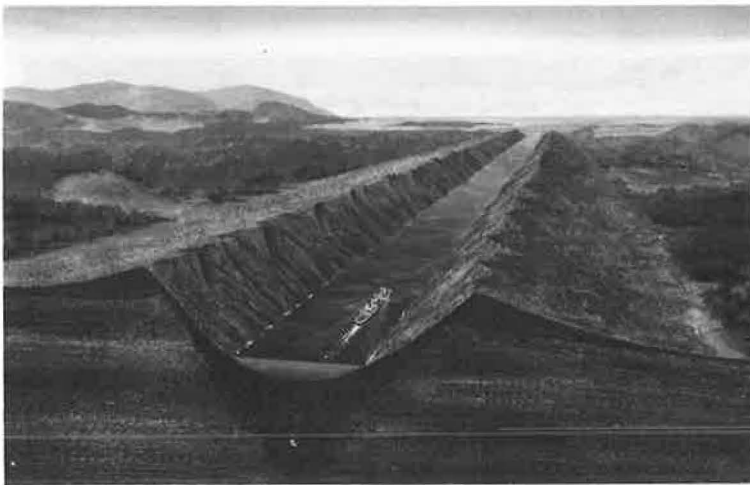
Figure 20. Artist's sketch of a nuclear-excavated canal through the Darien region of eastern Panama.
