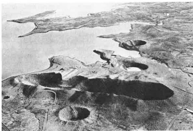
Figure 3. Pre-Gondola 20-ton single-charge craters and connecting row crater prior to execution of the reservoir connection experiment.
