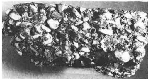
Figure 1. Field specimen showing stripping in actual pavement.
