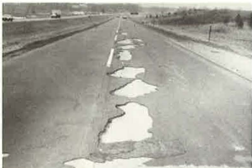
Figure 12. Synthetic bitumen and sand 1 year after construction.
