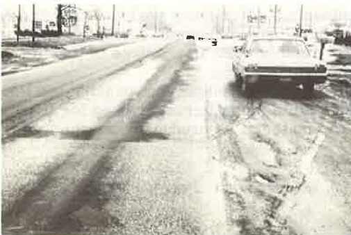
Figure 11. Crushed traprock 3 years after construction.
