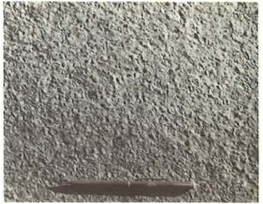
Figure 10. Close-up of beach-pebble surface 4 years after construction.
