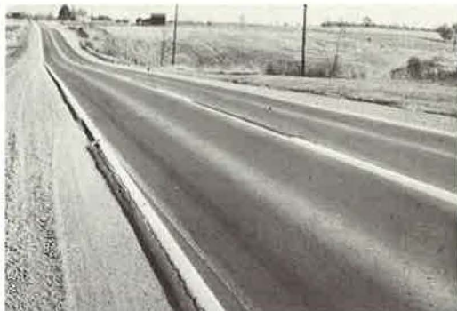
Figure 13. Sand-emulsion surface 4 years after construction.
