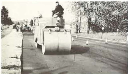
Figure 29. Rolling pavement after sand application.
