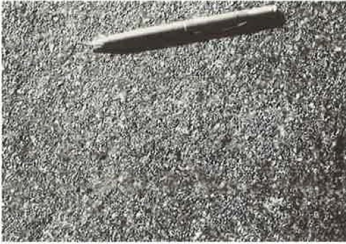
Figure 14. Close-up of sand-emulsion surface 4 years after construction.
