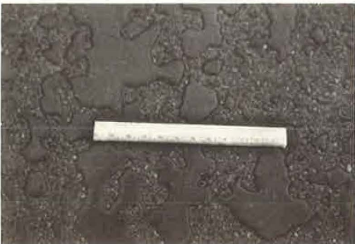
Figure 25. Close-up of fresh, oily, nonwetting bituminous surface after rain.
