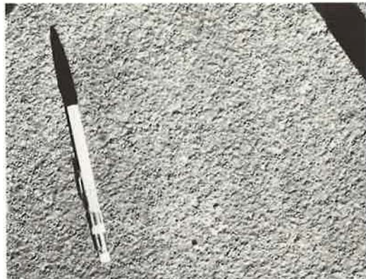
Figure 8. Close-up of quartzite surface 4 years after construction.
