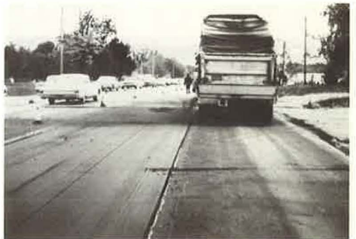
Figure 26. Spreading precoated sand on unrolled bituminous mat.
