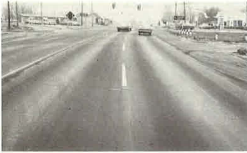
Figure 9. Crushed beach pebbles 3 years after construction.
