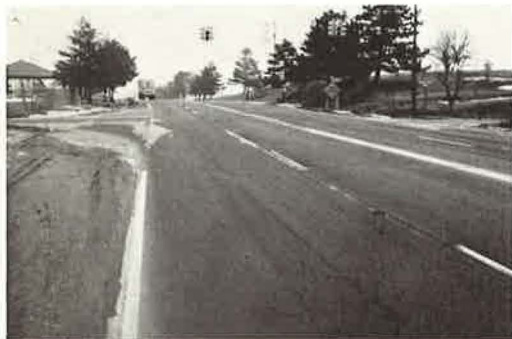
Figure 7. Crushed quartzite surface 3 years after construction.
