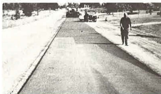
Figure 30. Pre-coated sand on mat of partly rolled surface.
