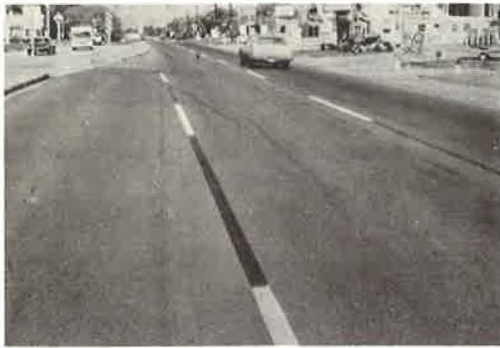
Figure 4. Crushed sandstone surface 4 years after construction.
