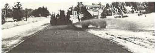
Figure 27. Spreading pre-coated sand without deflector (most of sand falls on shoulder).
