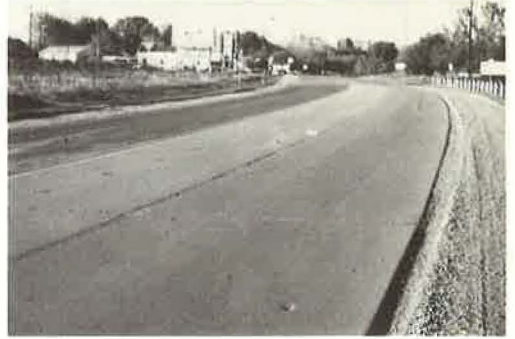
Figure 22. Sinopal-sand surface 4 years after construction.
