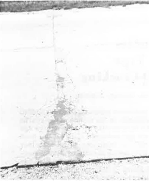
Figure 1. D-cracking along transverse joint of pavement.
