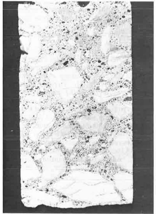
Figure 3. Vertical section of core taken through D-cracked pavement slab. Severe cracking in coarse aggregate particles extends into surrounding mortar.
