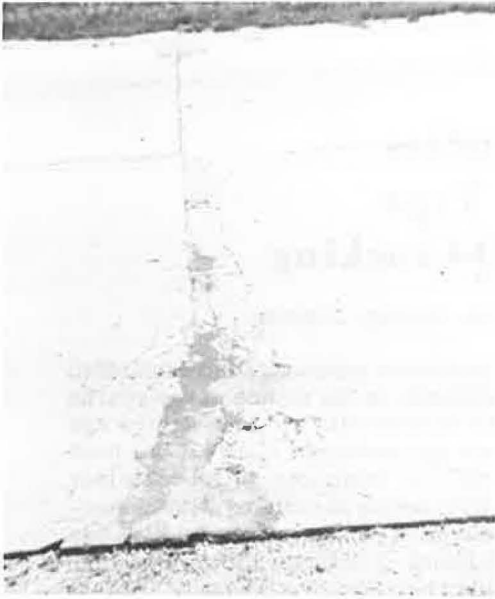
Figure 1. D-cracking along transverse joint of pavement.
