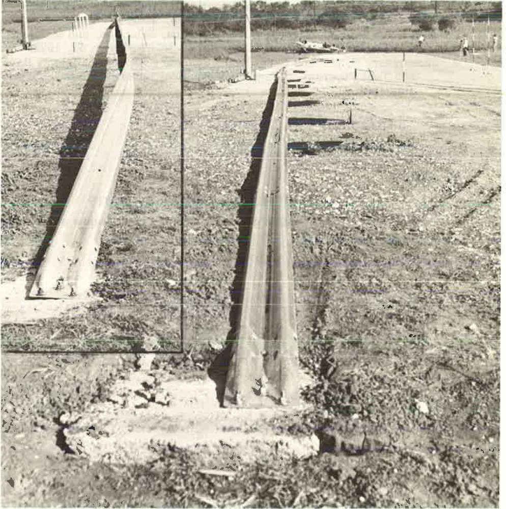
(a) Looking downstream (see insert for before test photograph)
