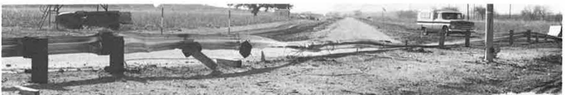
(d) View from behind rail after test
