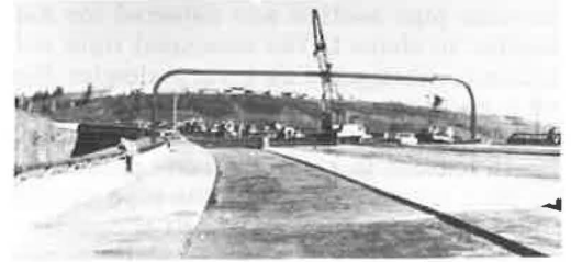
Figure 8. Simple three-piece erection—fast bolting-up operation (120-ft span; 20-in. pipe diameter).
