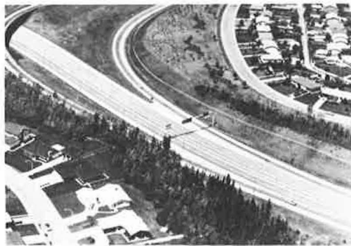
Figure 3. Long span provides clear gore area and flexibility of structure location (140-ft span; 20-in. pipe diameter).
