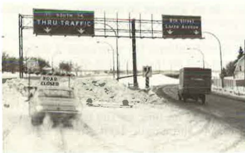
Figure 1. "Old style" overhead sign structure.
