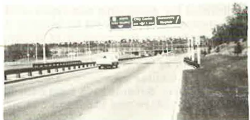
Figure 2. "New style" overhead sign structure (85-ft span; 14-in. pipe diameter).
