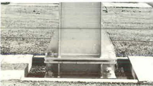
Figure 2. Details of breakaway base connection.
