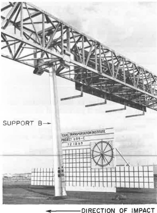
Figure 13. Impact area after Test C.
