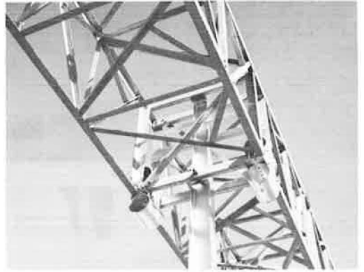
Figure 7. Load distributors at support B before Test B.
