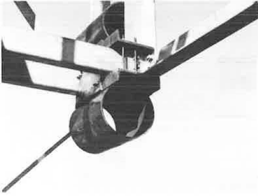
Figure 6. Load distributor bolted in place on lower truss chord at support A.
