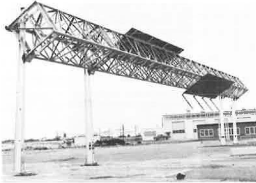
Figure 22. Condition of structure after Test H.
