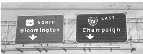
Figure 13. Conventional and louvered sign on overhead sign bridge.
