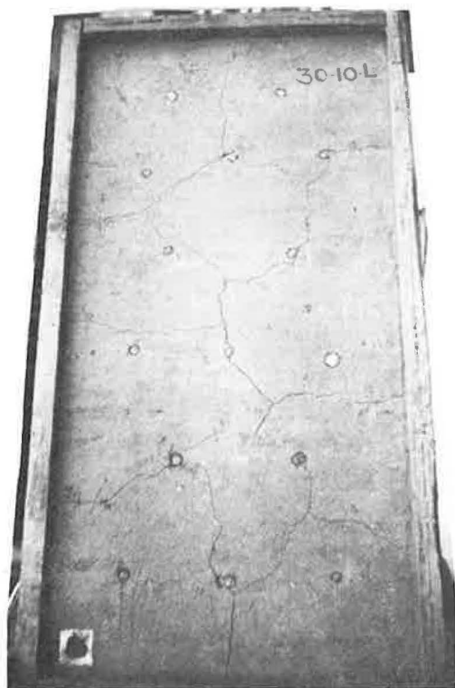
Figure 9. Crack pattern in gravel-embedded model for soil M30-10 (location of gravel shown by circles).
