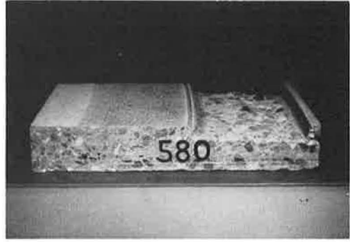
Figure 15. Four-inch portland cement concrete slab after test of 4 million tire passes (studded tires on right, tires without studs left of center, and original surface extreme left).
