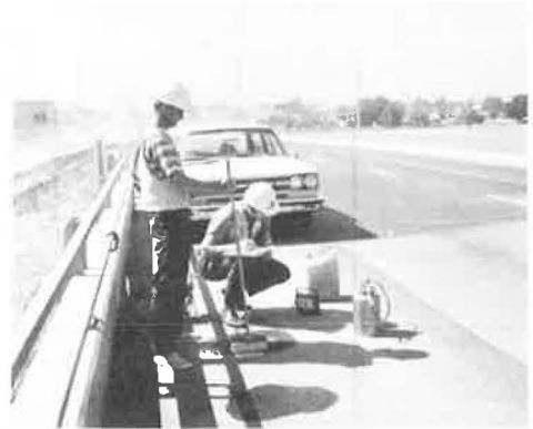
Figure 3. Measuring electrical resistance of bridge deck coating.
