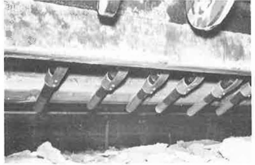
Figure 5. Internal vibrator mounted on paver.
