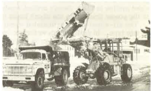
Figure 4. Wheel loader with side dump bucket, loading trucks.
