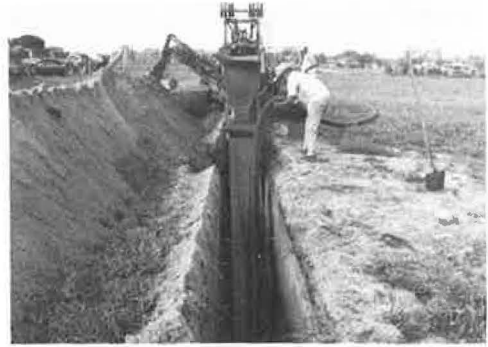
Figure 1. Installation of collector pipe and cloth A in subdrain system.
