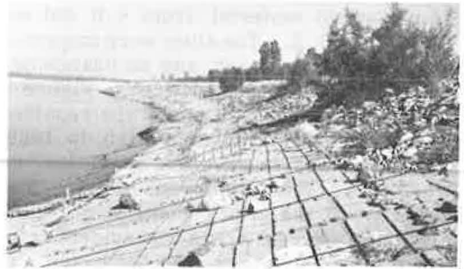
Figure 7. Island 63 revetted area underlaid with filter cloth (range 118+50).
