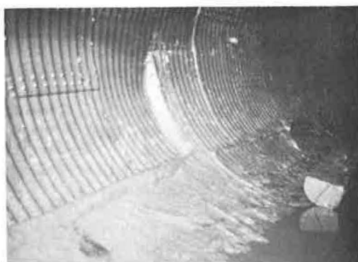
Figure 16. Failure of transverse joint in pipe shown in Figure 15.
