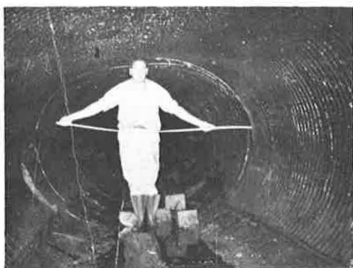
Figure 15. Excessive deflection of 84-in. storm sewer pipe.
