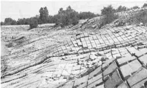
Figure 8. Island 63 revetted area underlaid with gravel bedding (range 123+00).
