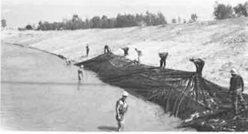
Figure 6. Placement of cloth B at Island 63.
