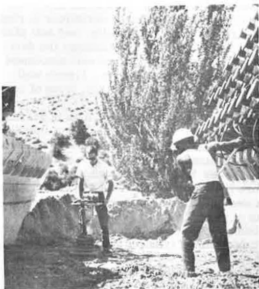
Figure 3. Technique for compacting the backfill in 1-ft lifts.
