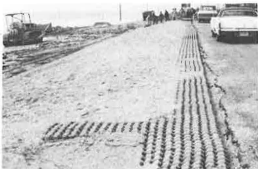
Figure 10. Louisiana Department of Highways test section (sand used as dry mortar).
