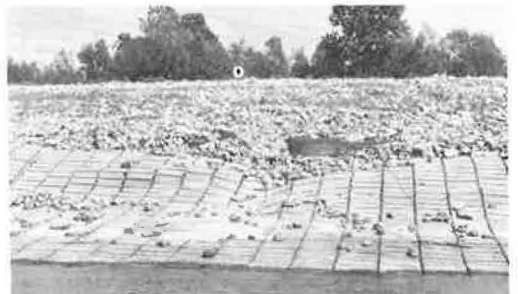
Figure 9. Island 63 bulged areas.
